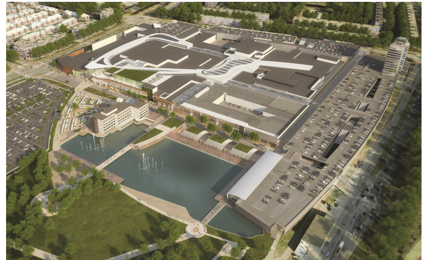
PROPOSED & RENOVATED ROOF FROM ABOVE
