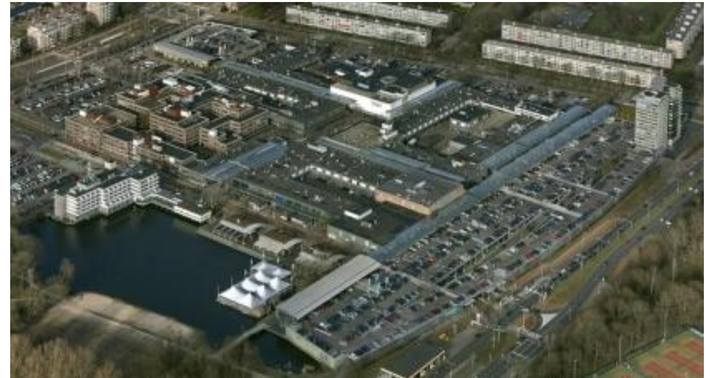
EXISTING ROOF FROM ABOVE
