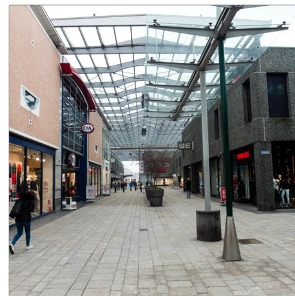
Mall of the Netherlands in aanbouw
