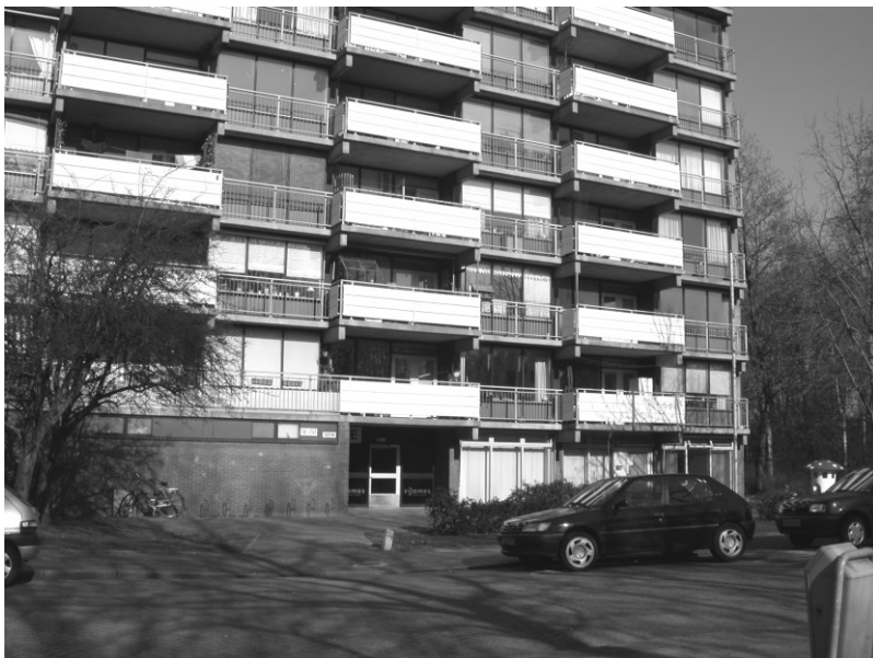
Foto 6: Entree complex De Tol
